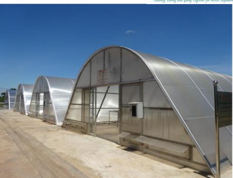
Drying using a greenhouse solar dryer
